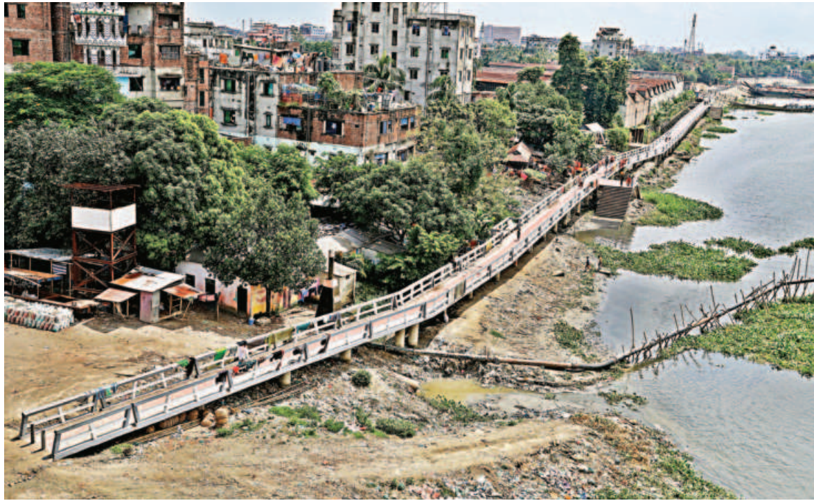
Around a decade ago, illegal establishments built by encroachers lined the banks of the Shitalakkhya. However, a government initiative to build a 52-km walkway on the sides of the Buriganga, Shitalakkhya and Balu rivers has changed the entire outlook of the spot as encroachers are now unable to grab the banks to build any structures. The photo was taken recently.
