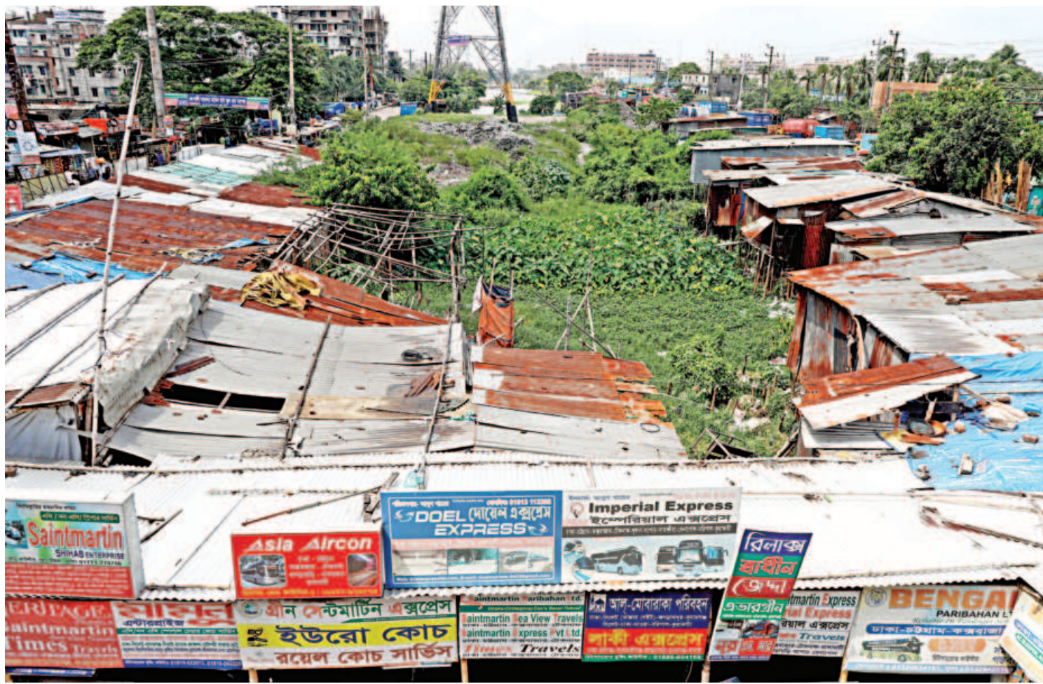
The DND canal along the Dhaka-Chattogram highway in Fatullah has been encroached upon by shops and different settlements. Such encroachment of waterbodies keeps going on unabated in different parts of the country, causing severe environmental and waterlogging issues. The photo was taken recently.
