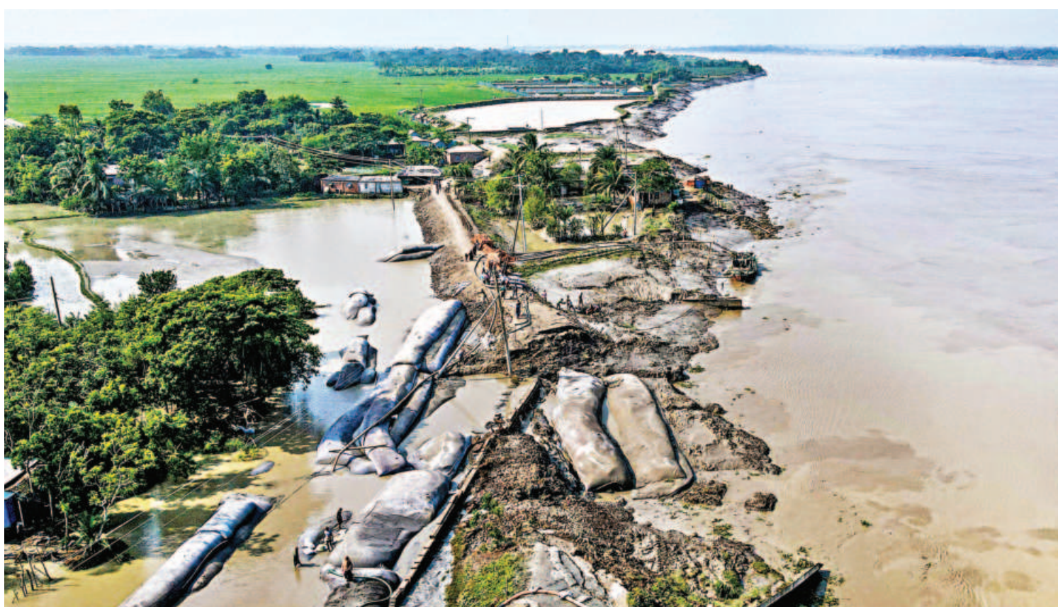
Several villages and thousands of bighas of cropland in Khulna's Dacope upazila have gone under water after tidal pressures broke down the Bhadra river's embankment there last Friday. The area is at further risk as coastal districts have been warned about the incoming Cyclone Dana, which is expected to make landfall between today afternoon and early tomorrow and impact the Sundarbans region. The photo was taken from Lokkhikhola village in the upazila recently.
