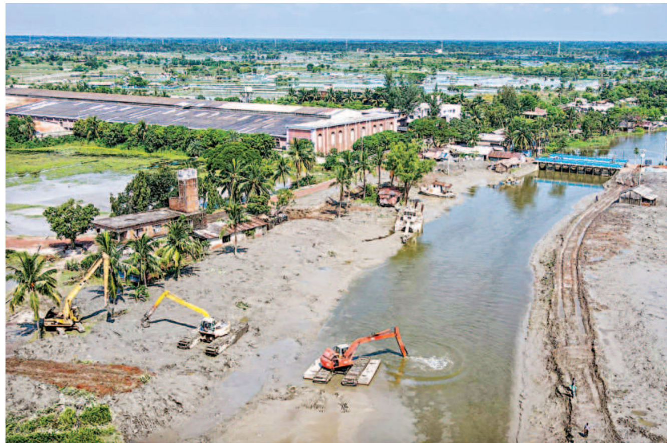
Silt accumulated near the Sholmari river sluice gate being removed by excavators. The river acts as the only means of water drainage for hundreds of villages in Khulna's Dumuria upazila. With so much silt near the gate, the villages have been facing intense waterlogging since the beginning of the monsoon. The photo was taken recently.
