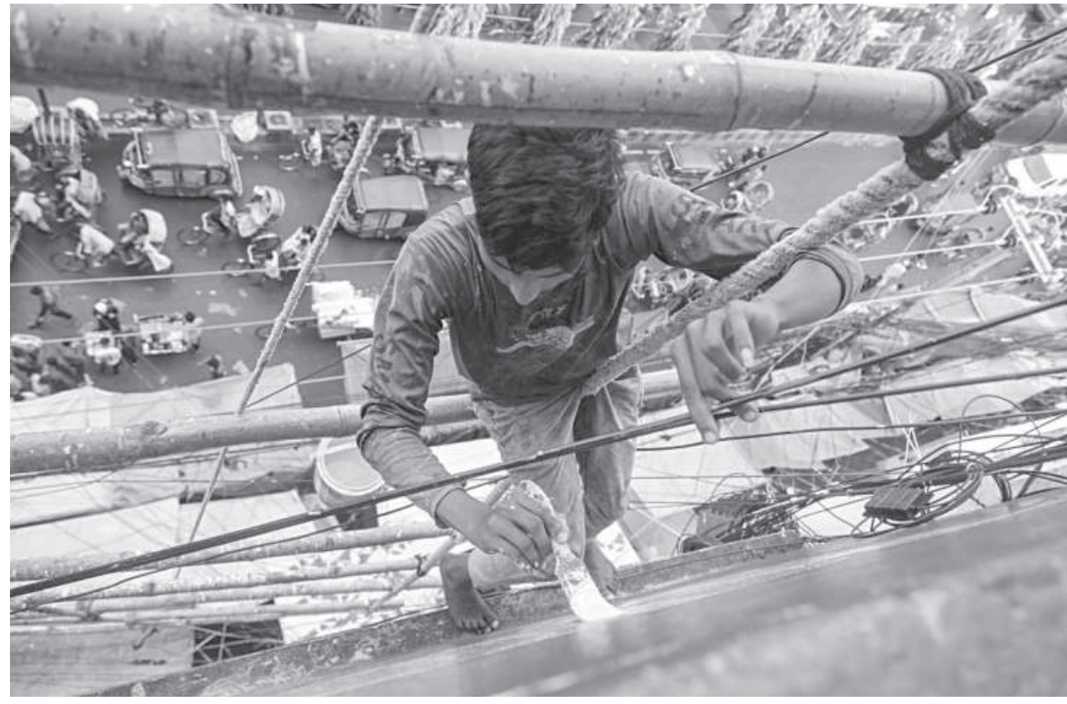
With no safety gear on, a construction worker paints a high-rise building in New Market area of Chattogram city yesterday. While deaths and injuries of such workers are common occurrences in the city and elsewhere, no substantial measures are visible in ensuring their occupational safety.
