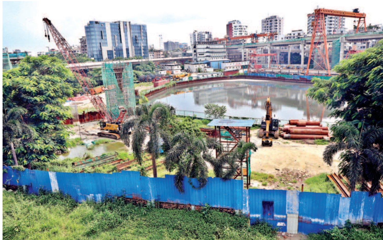
Large pillars and scaffolding rise from what was once a part of Hatirjheel. Over 10 acres of the waterbody has been filled with sand as part of the Dhaka Elevated Expressway. Cranes, excavators, and now temporary offices occupy the site. The place has been cordoned off with barricades. Authorities claim the filling was necessary to construct 41 pillars for the expressway, but environmentalists warn this could exacerbate the city's waterlogging woes. The photos were taken yesterday.
