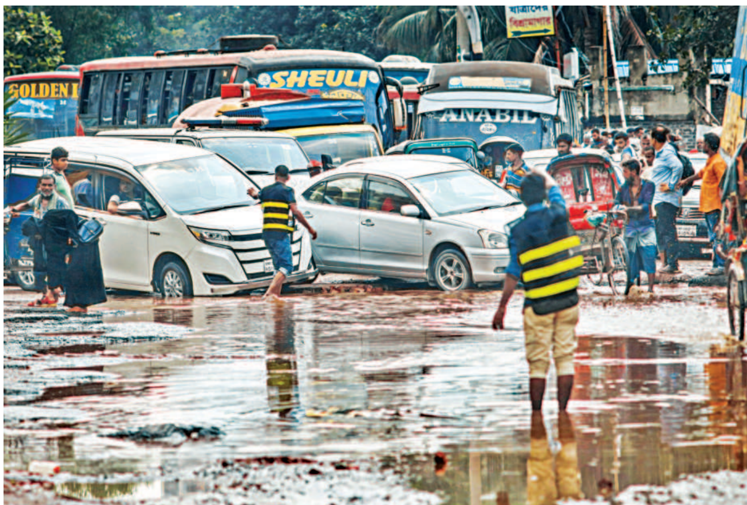
Vehicles navigate a crater-like pothole-ridden road in Kamalapur area in the capital yesterday. The poor condition of the street worsened following the recent rains. Breakdowns have become common on this patch of the road that often leads to congestion.
