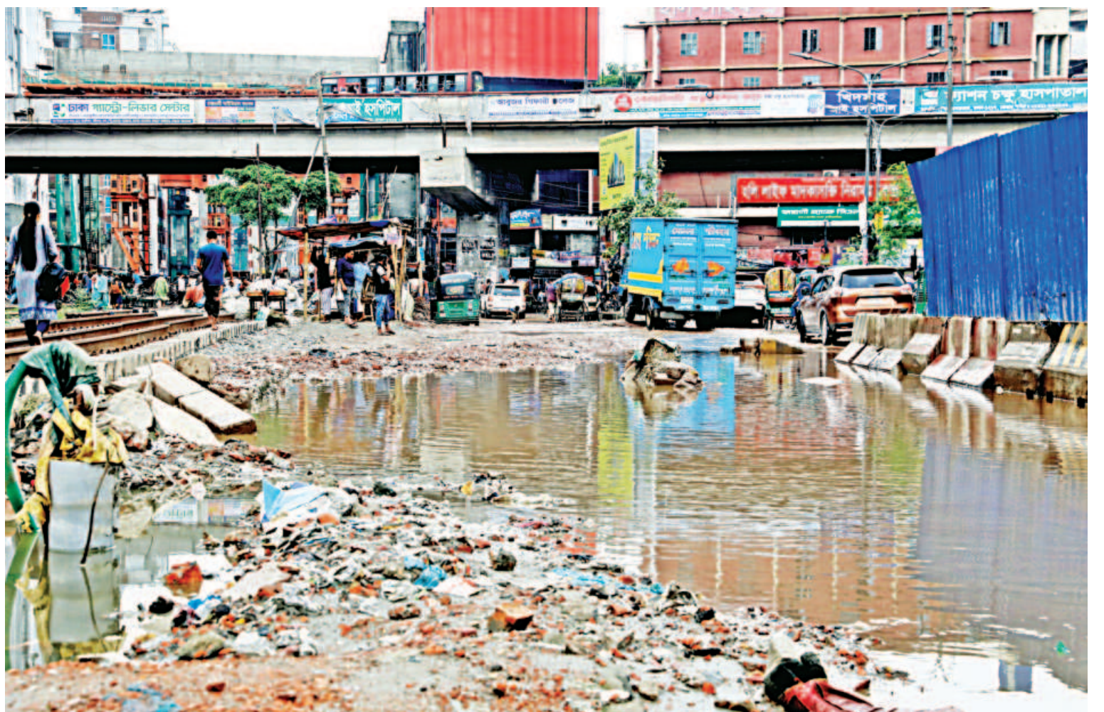
This road in Dhaka's Malibagh area remains waterlogged and littered with debris after rainfall, a recurring issue that brings daily hardship to pedestrians and vehicles alike. The photo was taken yesterday.
