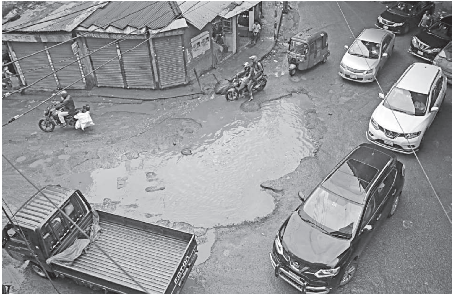
Just like this road near Joy Kali Mondir, many of Dhaka roads become unusable after just half a day of rain. Potholes form and water clogs the streets, as poor drainage fails to adequately address the issue. The photo was taken yesterday.
