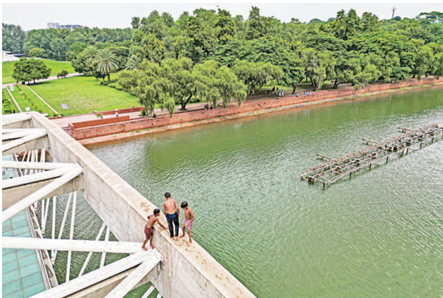
It's all fun and games until something goes wrong. As these children climb to the apex of the bridge at Crescent Lake in Chandrima Uddyan, a slight misstep could lead to a dangerous fall. The photo was taken recently.
