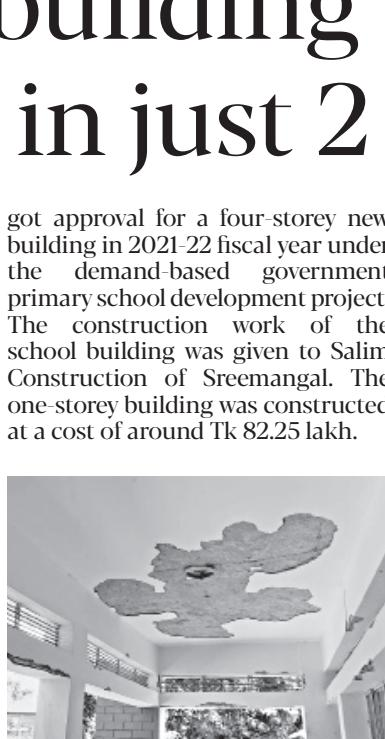
However, within two years of construction, cracks have appeared in the structure while plasters are getting removed in different places.
