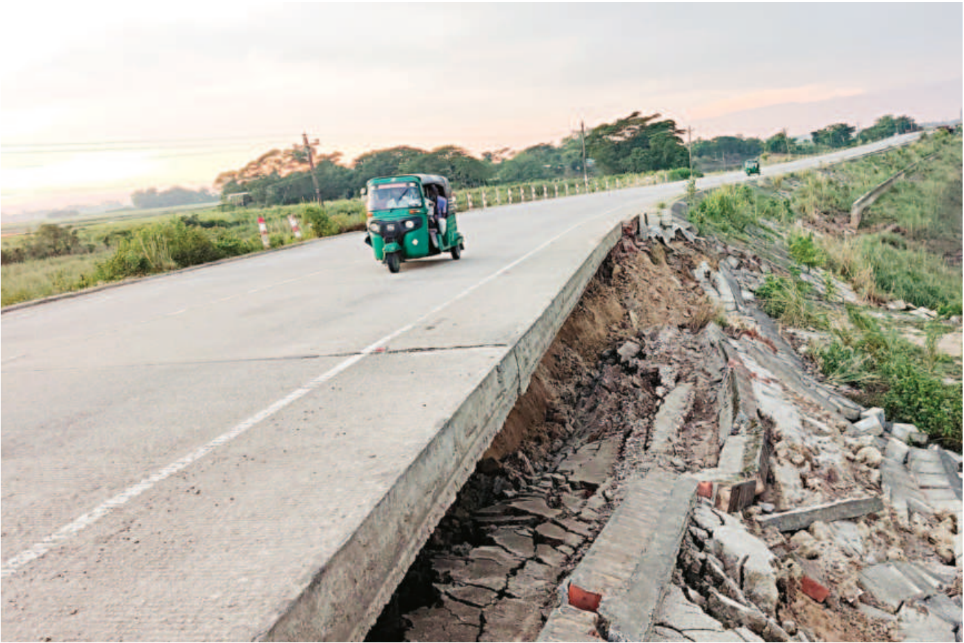
Soil beneath the Sylhet-Bholaganj highway has subsided, putting the road and vehicles travelling on it at risk. The photo was taken in High-tech Park area of Companiganj upazila on Monday.
