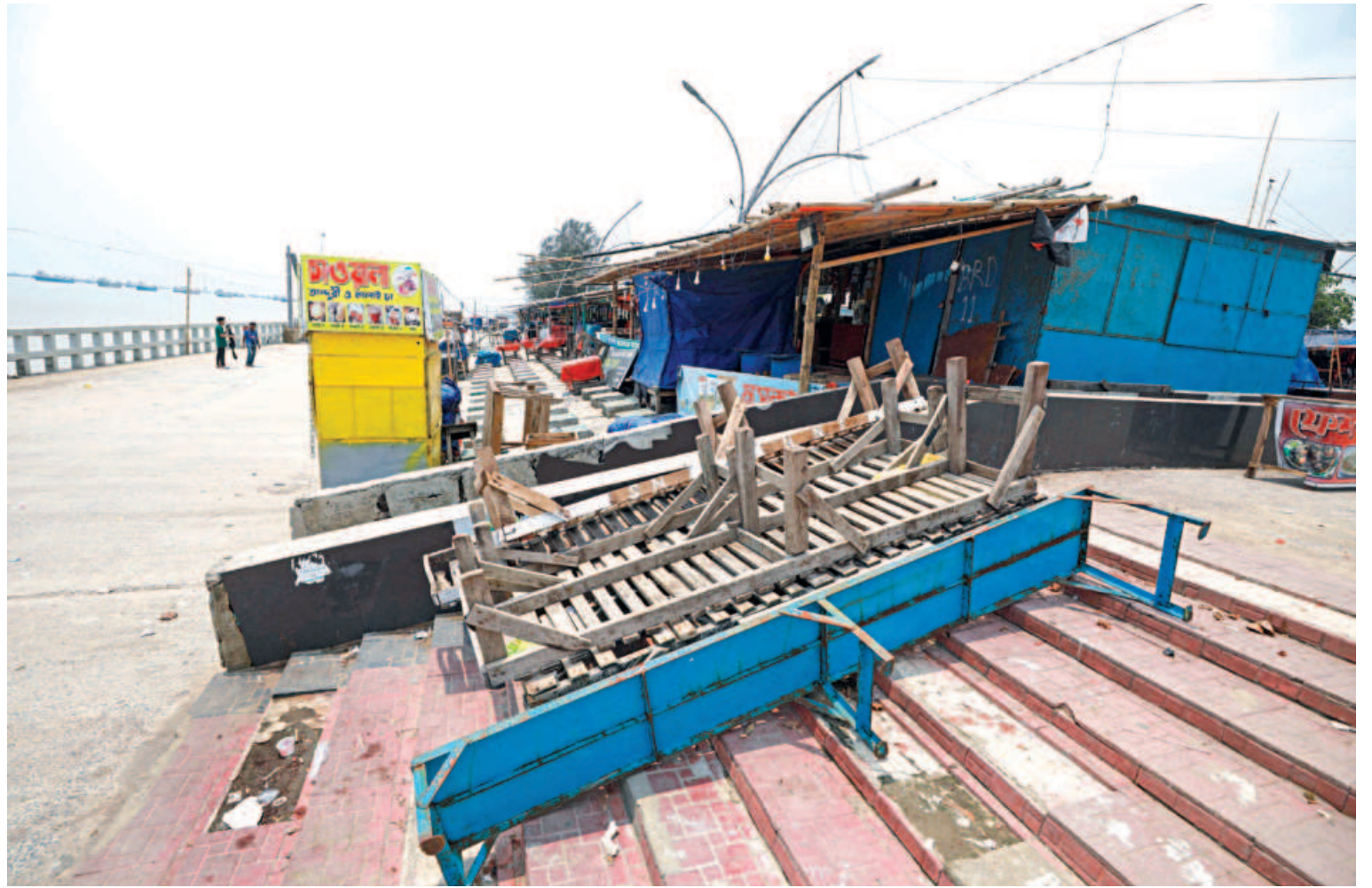
Illegal structures like restaurants, clothing stalls and souvenir shops keep sprouting along the seaside of Patenga beach in the port city. Syndicates charge these shops Tk 200-400 each day to allow them to continue their operations.
