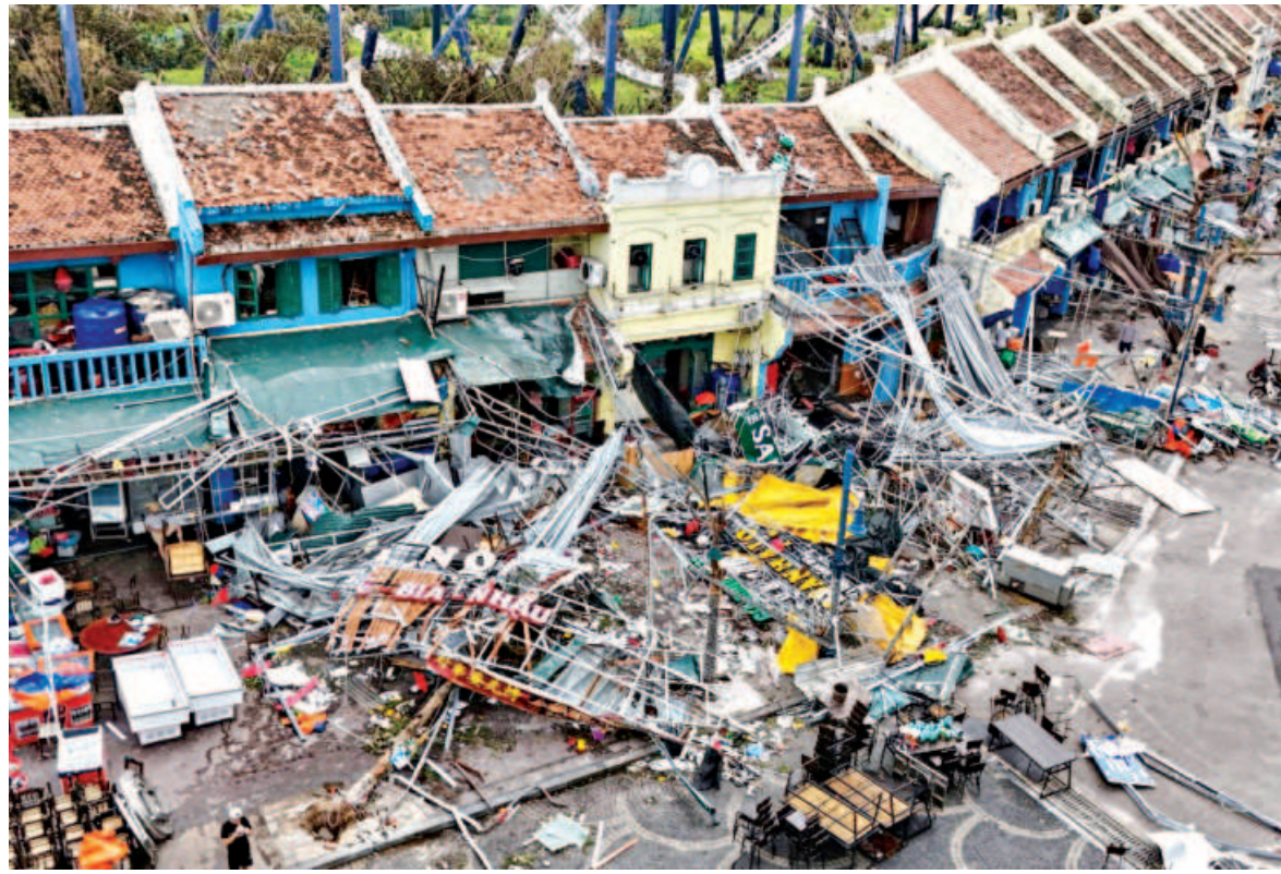
This aerial picture shows damaged buildings and debris on a street after Super Typhoon Yagi hit Ha Long, in Quang Ninh province of Vietnam yesterday.
