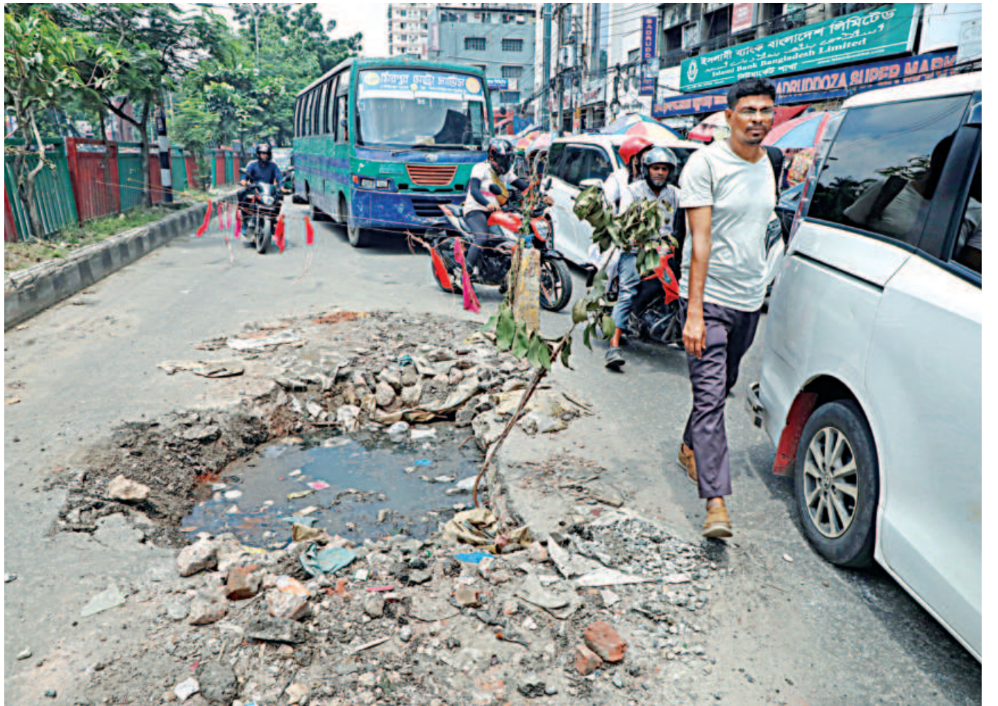
Amid the daily chaos of Mirpur Road, a large pothole filled with water near Dhaka College stands as a silent hazard. Marked but unfenced, it forces vehicles and pedestrians to navigate a perilous path. The photo was taken yesterday.
