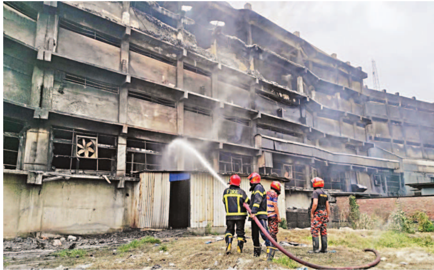
Firefighters spraying water to cool the Gazi Auto Tyres Factory in Narayanganj's Rugganj around 12:30pm yesterday. Though they could douse the fire on Tuesday, after a 32-hour hectic effort, small fires continue to flare up due to the extreme heat. The six-storey factory, owned by former Awami League minister Golam Dastagir Gazi, was set on fire by arsonists on Sunday night. PHOTO: SAURAV HOSSAIN SIAM
