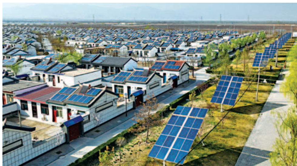
An aerial view shows residential buildings with roof-mounted photovoltaic solar panels in Yinchuan, in northwestern China's Ningxia region. In 2023, China accounted for more than half of the world's new wind and solar installations.
