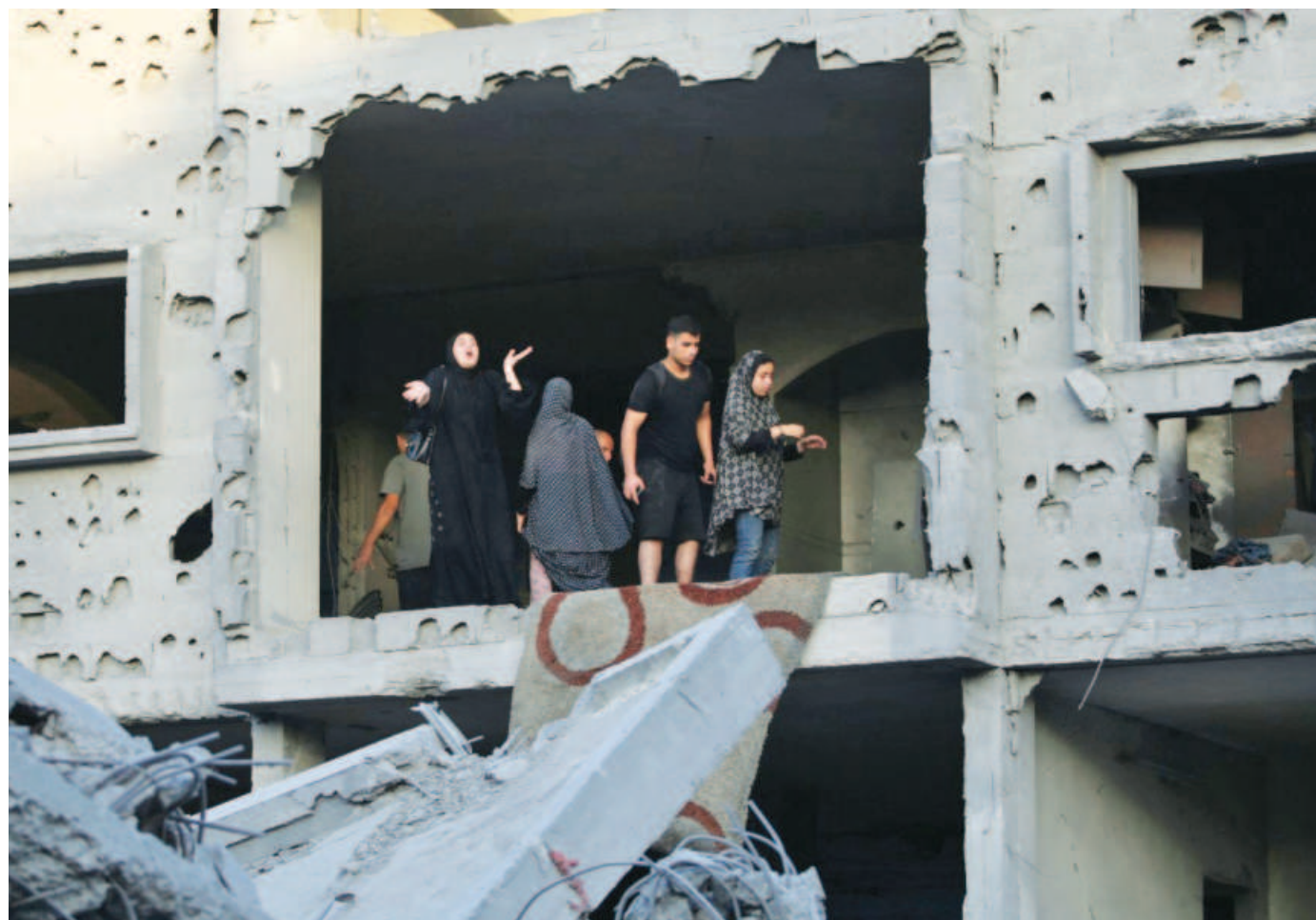
Palestinians stand on the balcony of a damaged flat in the vicinity of a building which was levelled by Israeli bombing in the Nuseirat refugee camp in the central Gaza Strip. The photo was taken on Thursday.
