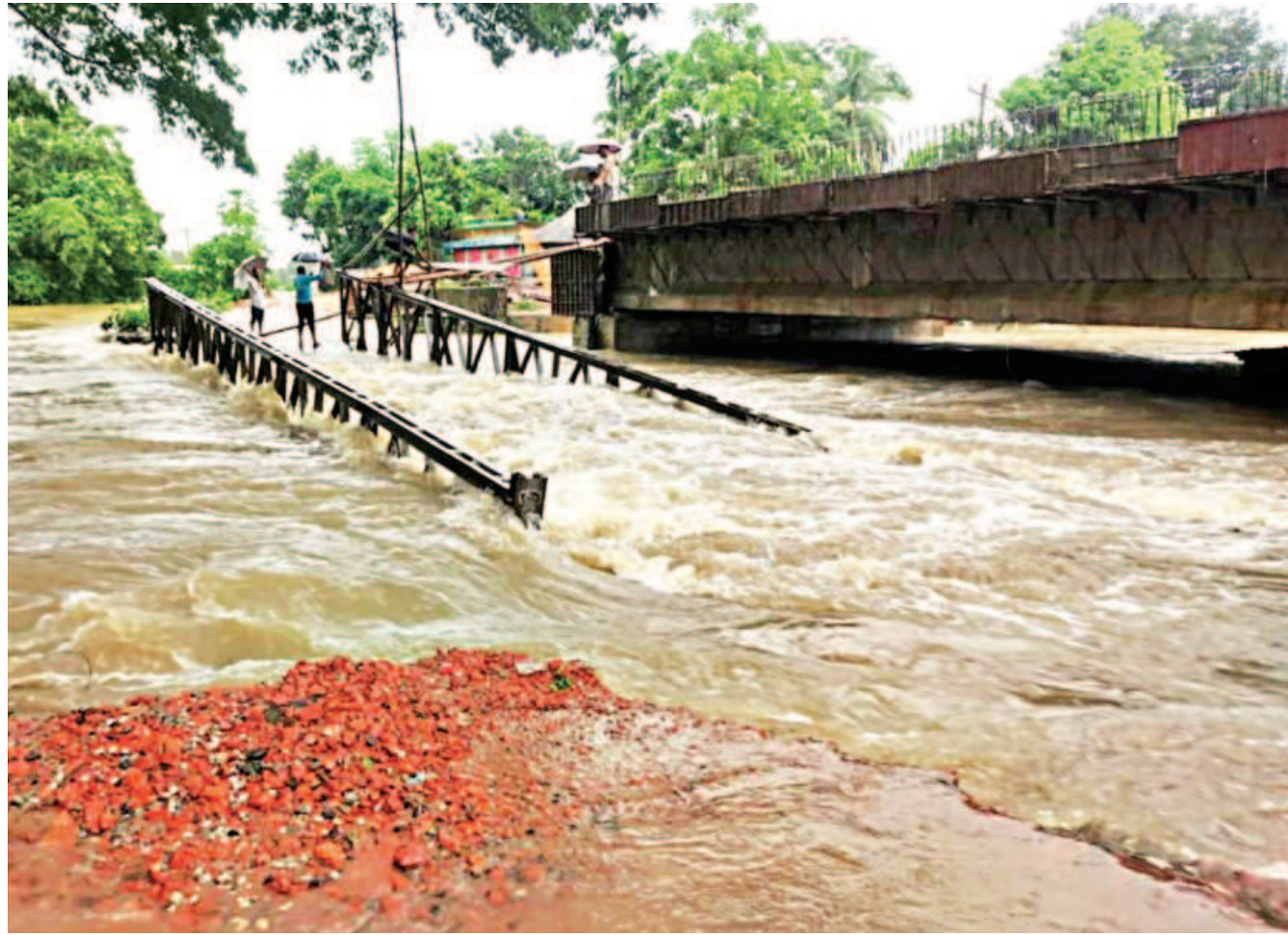
A Bailey bridge over the Kalundi canal on Akhaura-Agartala road collapsed yesterday morning due to onrush of water fed by downpours upstream. At least 15 villages of Brahmanbaria's Akhaura upazila and the Akhaura land port have been hit by floods. PHOTO: MASUK HRIDYO
