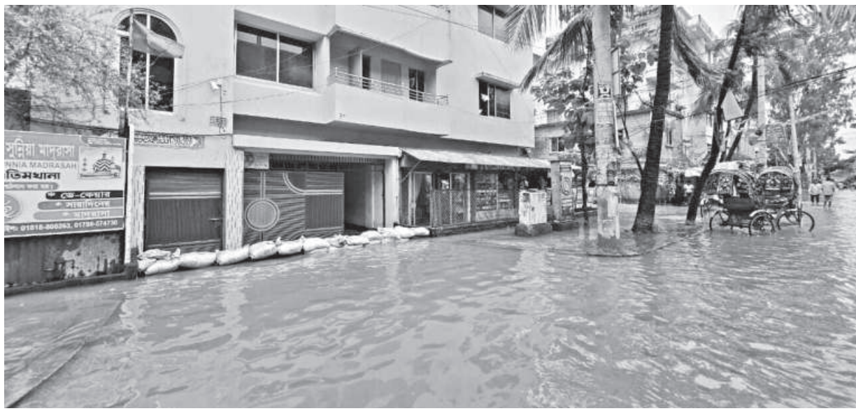
Persistent waterlogging in Chattogram highlights the city's struggle with uncleaned drains, amid political unrest and heavy rains, leaving residents in knee-deep water and disrupting daily commutes. PHOTO: COLLECTED
