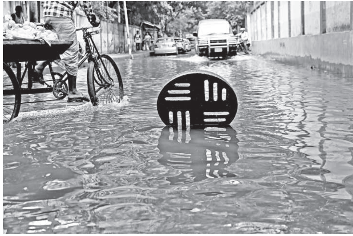
With an open manhole lurking underwater, vehicles ply a submerged road near Dhaka College. A moment of carelessness can lead to an accident. The photo was taken yesterday.
