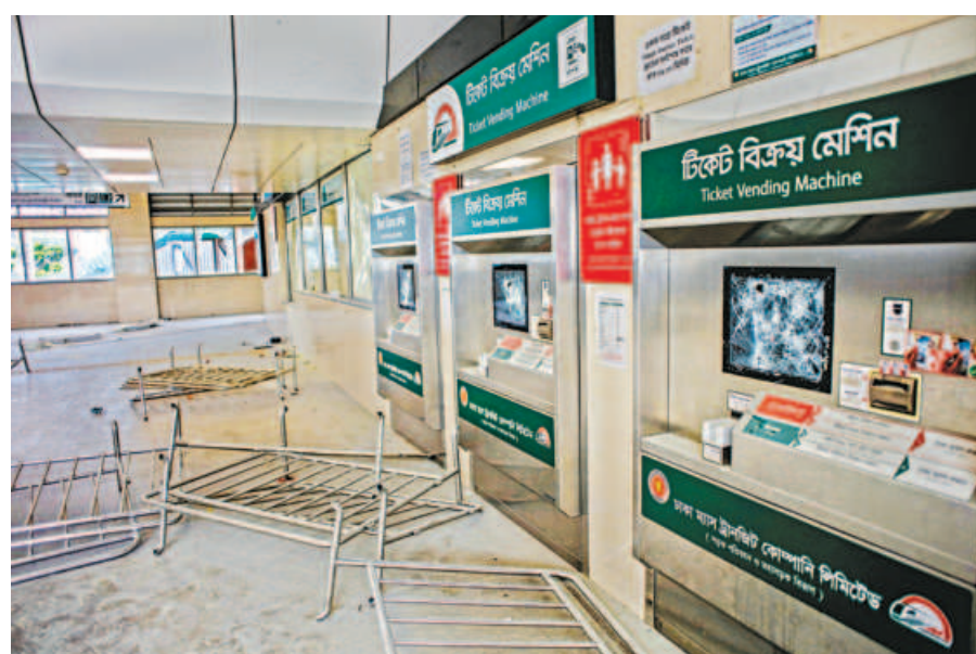
The ticket vending area at the station of Dhaka Metro Rail in the capital's Mirpur-10 was vandalised during the countrywide unrest on July 19. PHOTO: RASHED SHUMON
