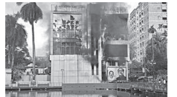
Annex Bhaban on Sadar Road in Barishal was set on fire on August 5.
