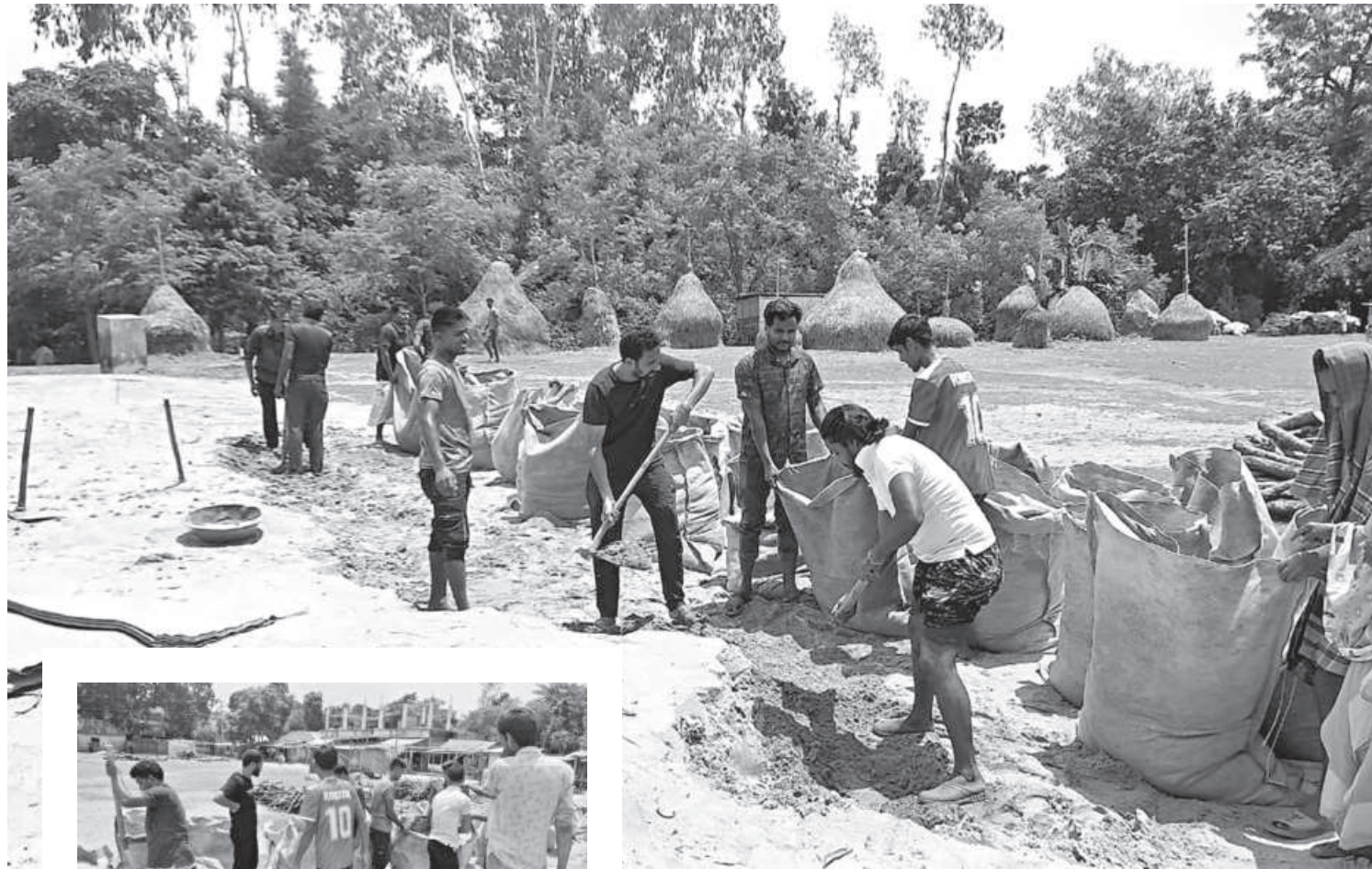
A group of students, along with locals, repairing a damaged road in Phulbari upazila of Kurigram yesterday. The road had sustained significant damage due to heavy rains two weeks back. The photo was taken near the Helipad area in Phulbari Sadar union.
