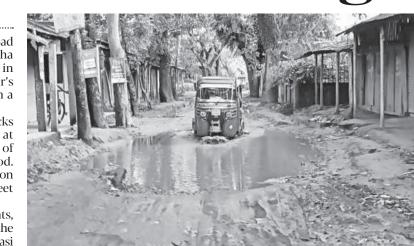
Jasim Uddin, a driver of CNGrun auto-rickshaw, said, "The road surface is severely damaged. The entire seven-kilometre stretch has hundreds of potholes of different shapes. Some are so wide and deep that whenever it rains, water accumulates in those potholes to resemble a ditch. Driving vehicles on the road has become very risky and turbulent, and accidents can happen any time."
