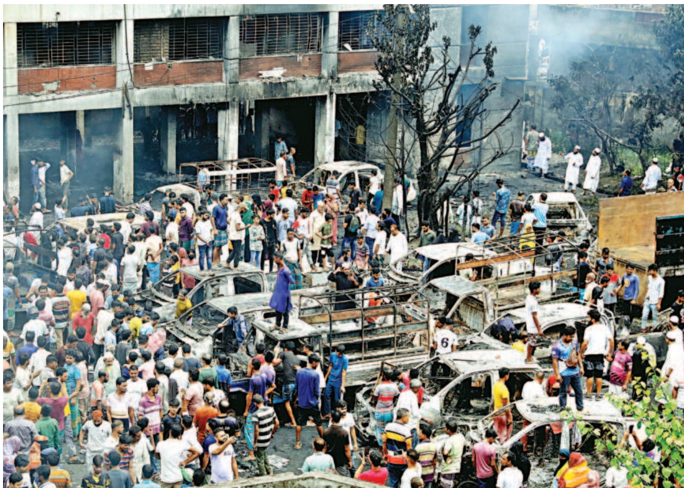
People looking at the damage done to Jatrabari Police Station, a day after a mob set it on fire. Several vehicles, furniture and valuables were burnt in the arson attack. There were no law enforcers at the facility yesterday.
