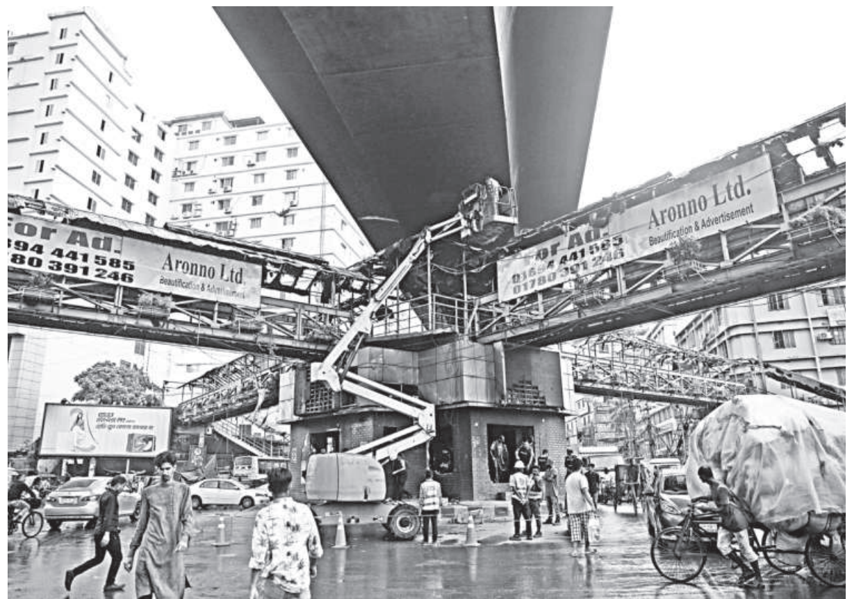
Employees of Dhaka Mass Transit Company Limited inspect a section of the metro rail at the Mirpur 10 intersection area yesterday. During the recent unrest in the country, this foot-bridge was set on fire, which is why the DMTCL is checking to see if any damage occurred to the metro rail.
