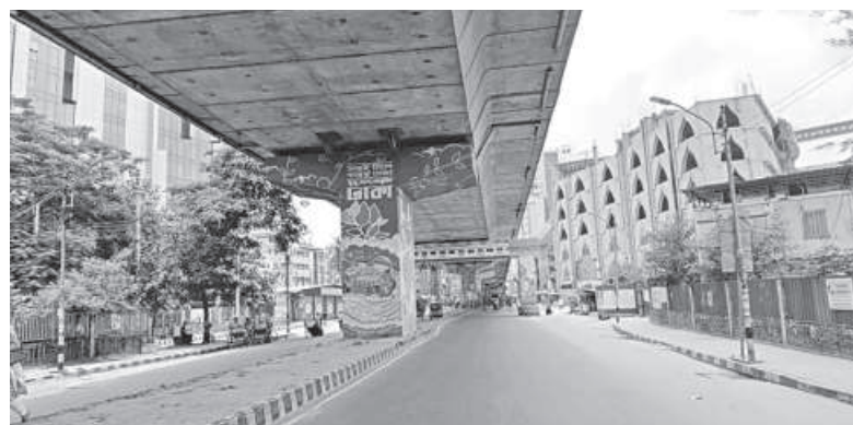
A road in Moghbazar.
