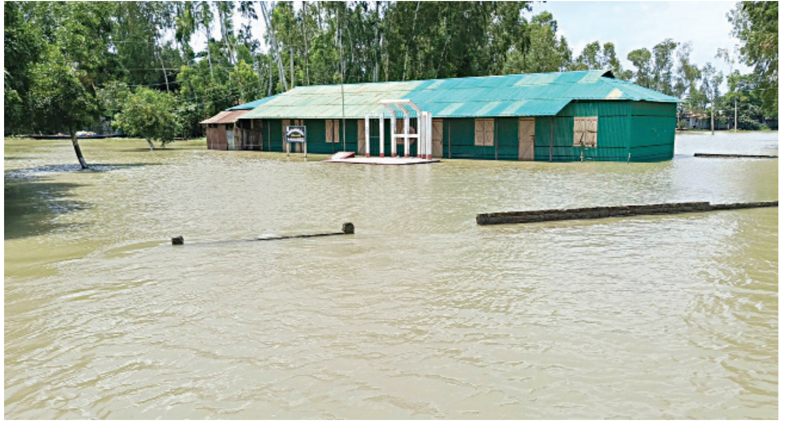
The Patrakhata Feichka Government Primary School in Putimari char area of Kurigram's Chilmari upazila has been submerged for the past one week. With the Brahmaputra still flowing above the danger level, at least 80 homesteads, along with croplands, remain flooded in this area. The photo was taken yesterday.
