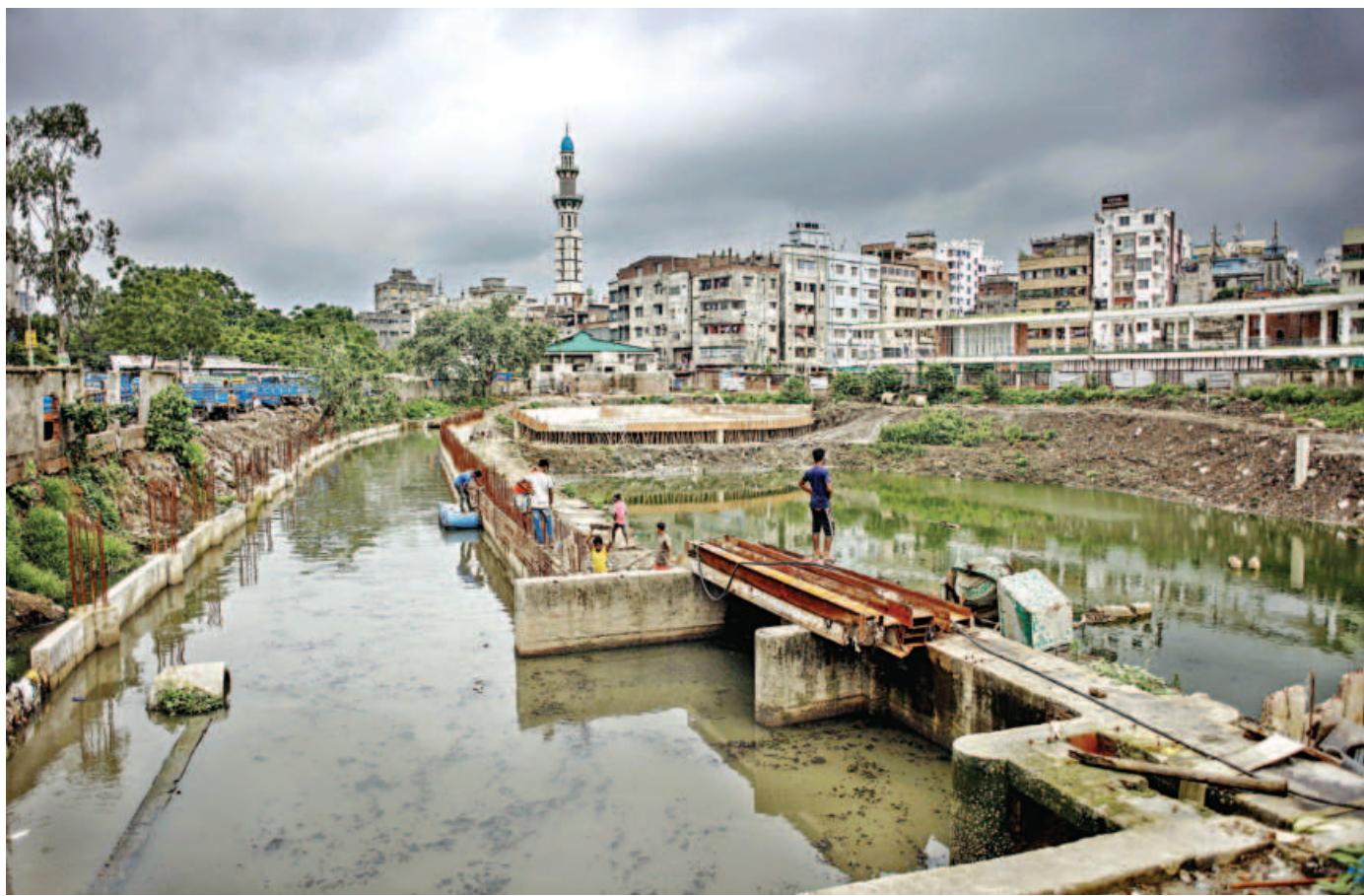
The capital's Dholaiakhal, which has been in a sorry state for years, is going to change. Dhaka South City Corporation has taken up a project to build two amphitheatres, walkways, bicycle lanes, and improve the waterbody on five acres. PHOTO: RASHED SHUMON
