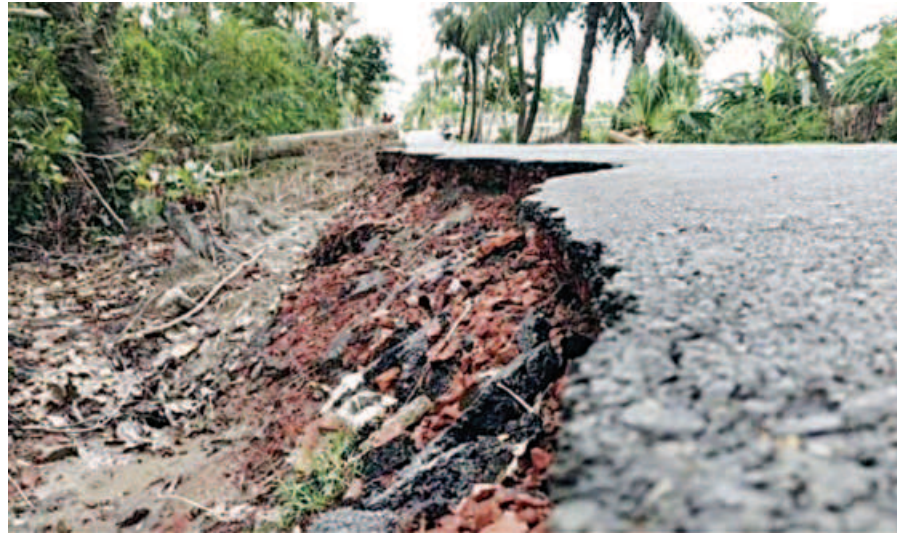
Like this one, several cracks have developed on this newly constructed road in Barguna's Patharghata upazila even before handing over the project.
