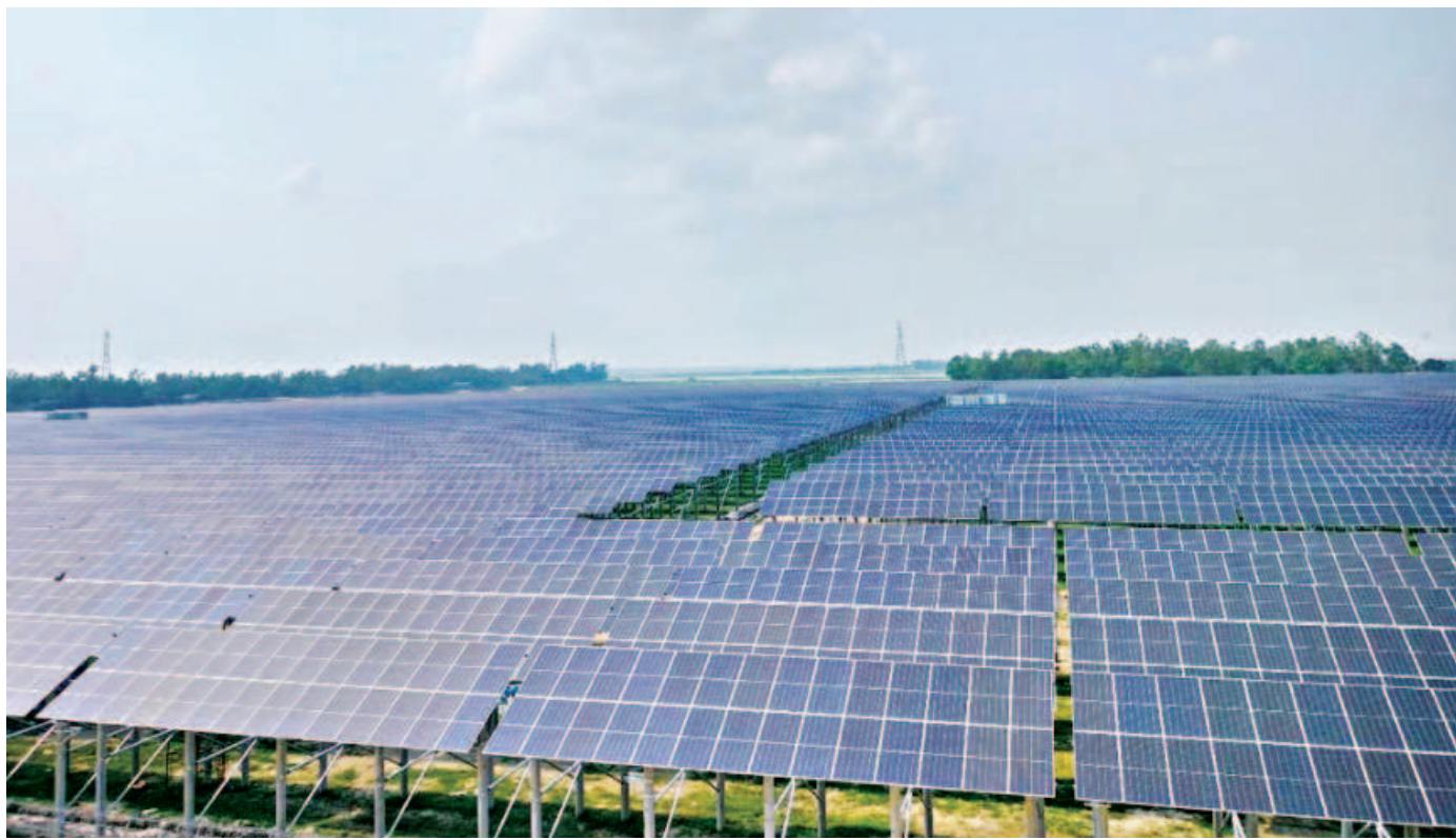
An array of solar panels at the Sirajganj 68MW Solar Park in Soyadabad near Bangabandhu Bridge. A total of 1.56 lakh solar panels have been set up there. The photo was taken recently.
