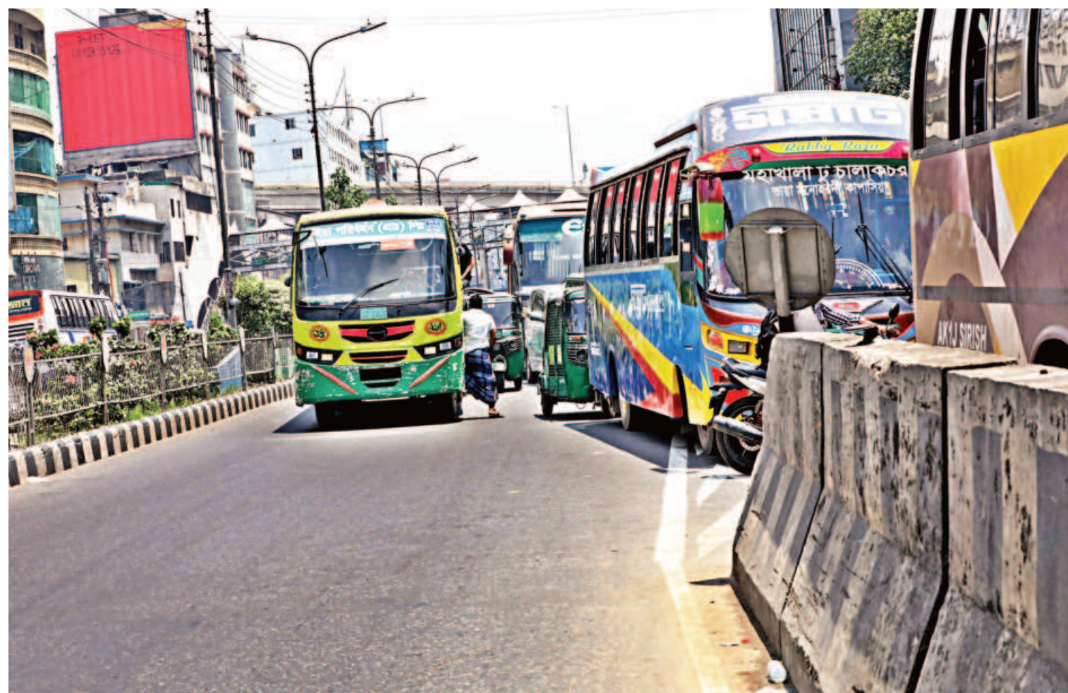
Buses heading towards Mohakhali intersection block the ramp of Mohakhali Flyover, not in picture, in the capital's Chairmanbari area, leading to tailbacks on this busy road. The photo was taken around noon yesterday.
