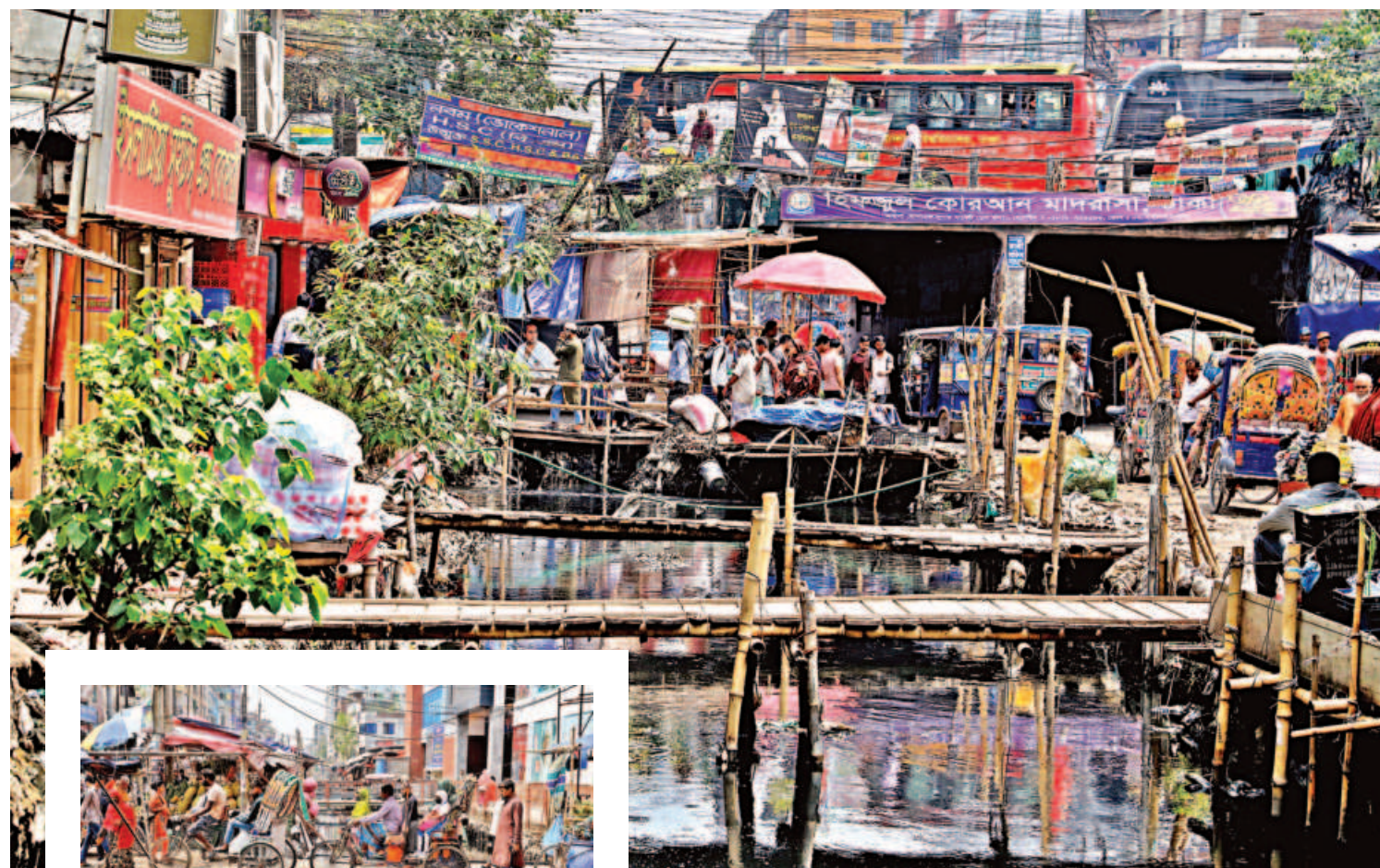
These makeshift bridges set up by locals over a canal are being traversed daily. Some of them are even being used by battery-run rickshaws. This sort of temporary solution pose a risk to pedestrians as they could collapse at any moment. The photo was taken in the Jatrabari area recently.
