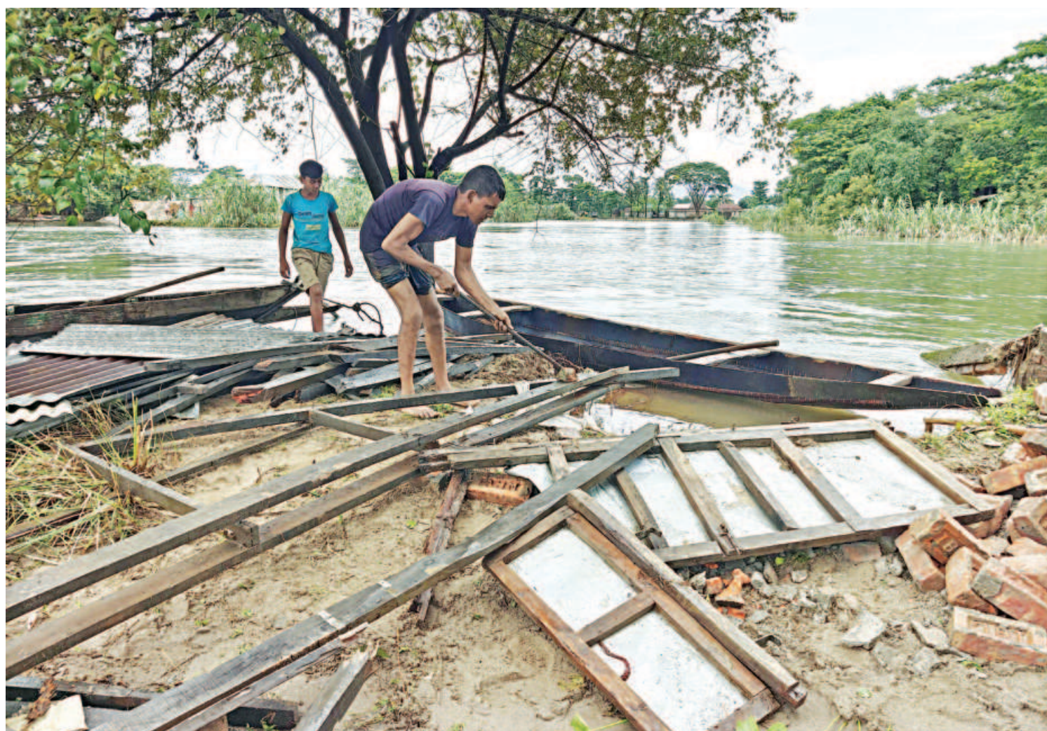
Amir Ali and his brother were seen clearing out the ruins of their broken house in Bordeo village in Pashchim Islampur union of Sylhet's Companiganj upazila on Saturday. Many houses in the upazila were damaged or broken beyond repair due to the recent floods that hit the Sylhet division.
