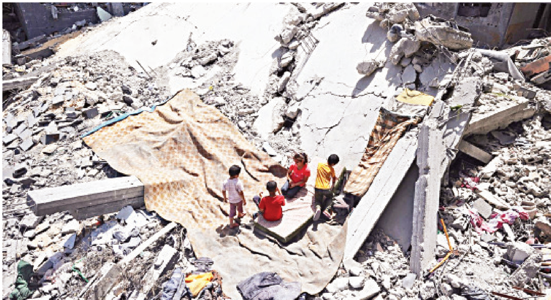
Palestinian children play on the site of a destroyed building in the Nuseirat refugee camp, in the central Gaza Strip yesterday. As Muslims worldwide prepare to mark Eid-ul-Azha starting today, Gazans lamented the shortages of essential goods and the lack of an Eid spirit amid Israeli bombardment. PHOTO: AFP
