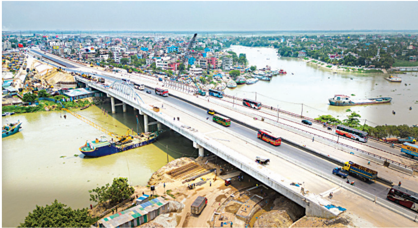
The new six-lane bridge adjacent to the existing four-lane Amin Bazar Bridge is now fully open to traffic. Two lanes of the bridge were opened in April and the remaining four on Wednesday. The bridge is expected to ease traffic congestion in the Gabtoli-Amin Bazar area. The photo was taken on Wednesday.
