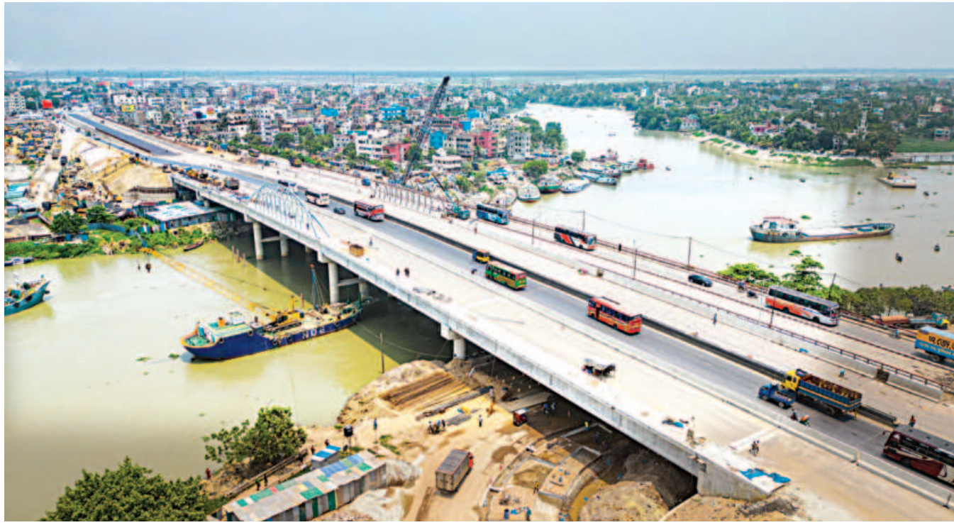
The new six-lane bridge adjacent to the existing four-lane Amin Bazar Bridge is now fully open to traffic. Two lanes of the bridge were opened in April and the remaining four on Wednesday. The bridge is expected to ease traffic congestion in the Gabtoli-Amin Bazar area. The photo was taken on Wednesday.
