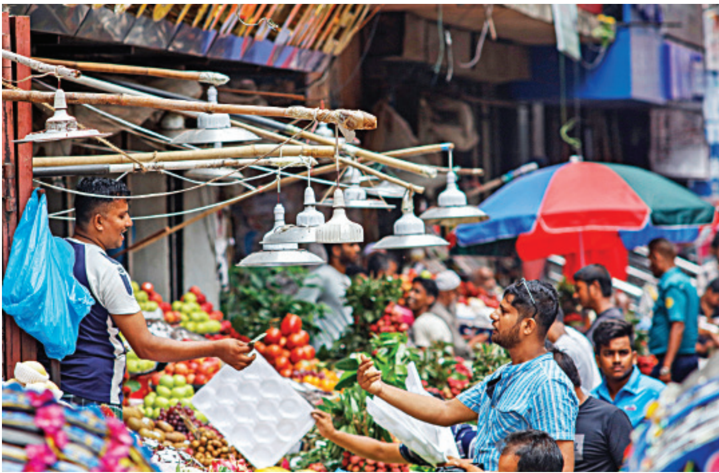
These illegally set up power connections on footpaths not only cause losses but also consumes a chunk of the available power in the capital. Despite load shedding being a constant menace in the city, such activities continue unabated. The photo was taken in the Purana Paltan area recently.
