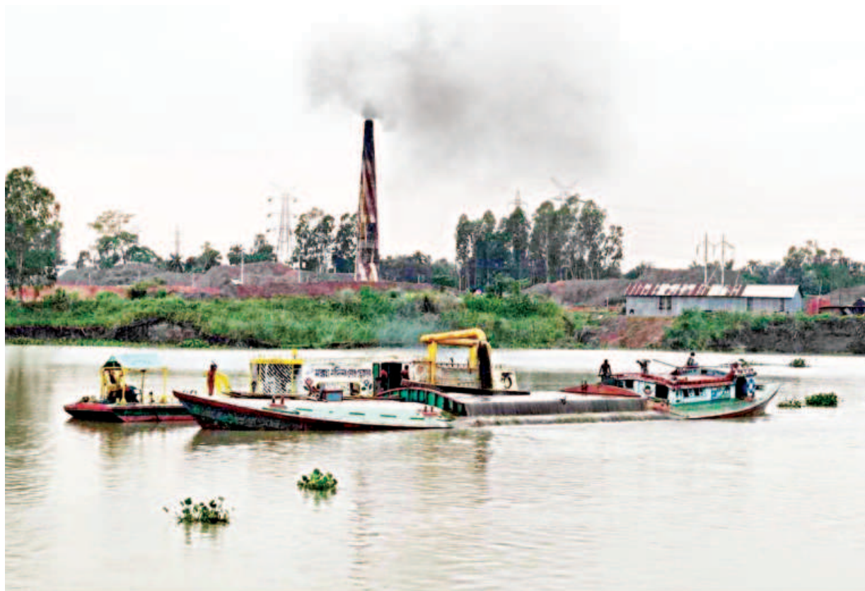
Dredgers being used to extract sand from the Bangshi river in Tangail's Mirzapur upazila. This illegal activity has also exacerbated the erosion threat, inset.
