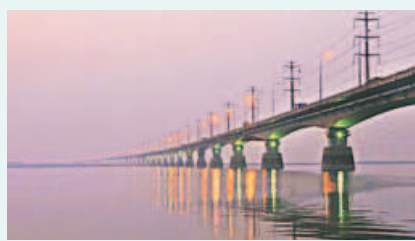
The Bangladesh Bridge Authority will replace all pot bearings on the 4.8km Bangabandhu Bridge at a cost of Tk 128.47 crores, marking the largest maintenance effort since its opening 26 years ago.
