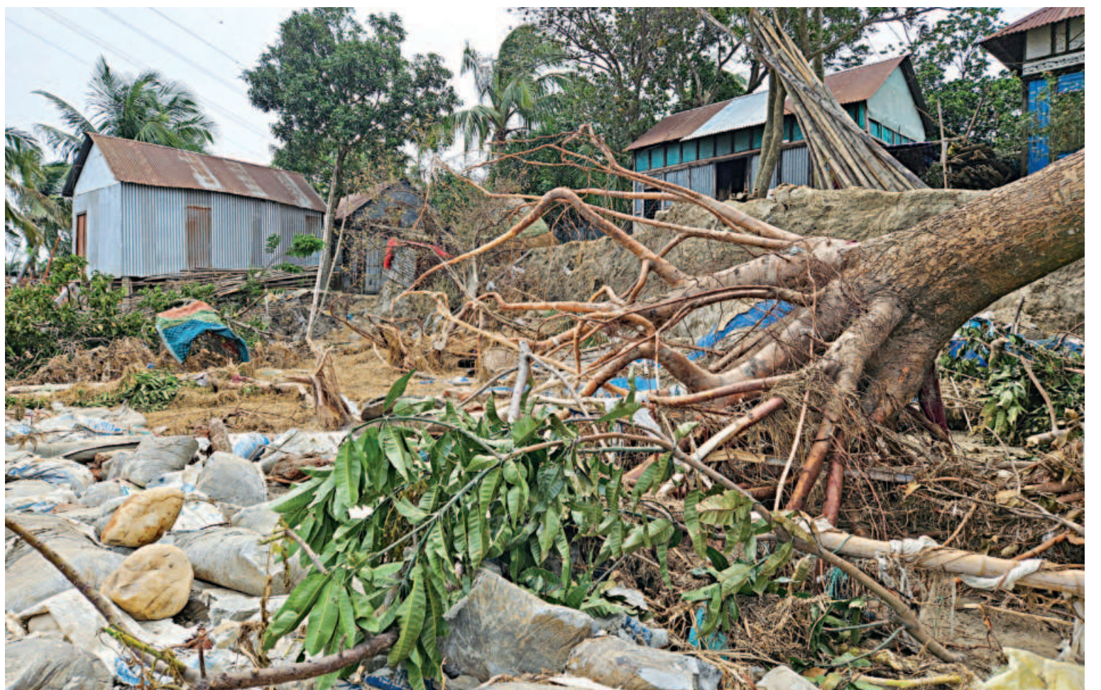
In the wake of Cyclone Remal, at least 16 tin-shed houses were destroyed and 10 damaged in Char Balaki village of Gazaria upazila, near the Meghna River in Munshiganj. Trees have fallen over, roads have been damaged and numerous livestock have been lost as well. Even four days later, locals are still repairing their damaged homes.
