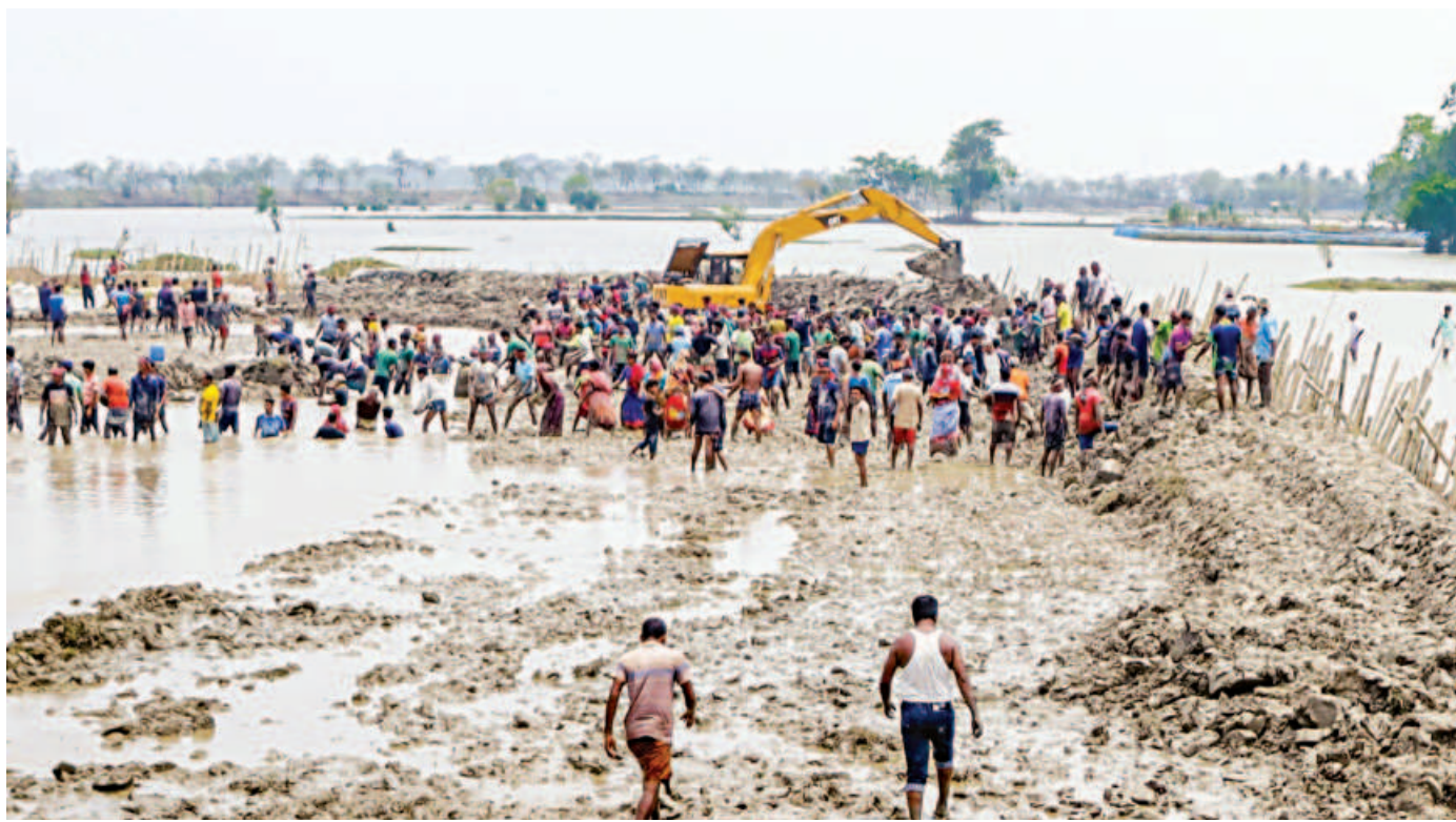
Locals of several villages were building an earthfill dam on the Bhadra river using a rented excavator yesterday, before beginning repair work of the broken embankment in Deluti union of Khulna's Paikgachha upazila. They have taken it upon themselves to fix the protective structure as there is no government initiative in sight as yet. The embankment breach has caused damages to farmlands, houses, animals and trees across the upazila.
