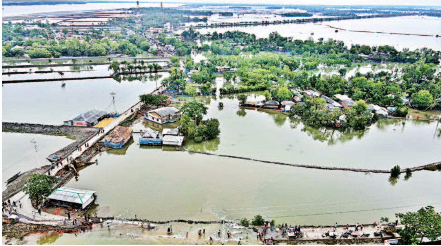
THE AFTERMATH ... Soldana and other neighbouring villages in Khulna's Paikgachha upazila have gone under water after Cyclone Remal breached a Shiba river embankment, washing away a large number of crab and shrimp farms. The water has also engulfed a part of a road that was vital for the villagers, further adding to their woes. Thousands of people have been affected by the flooding there. The photo was taken yesterday. More photos on P2.
