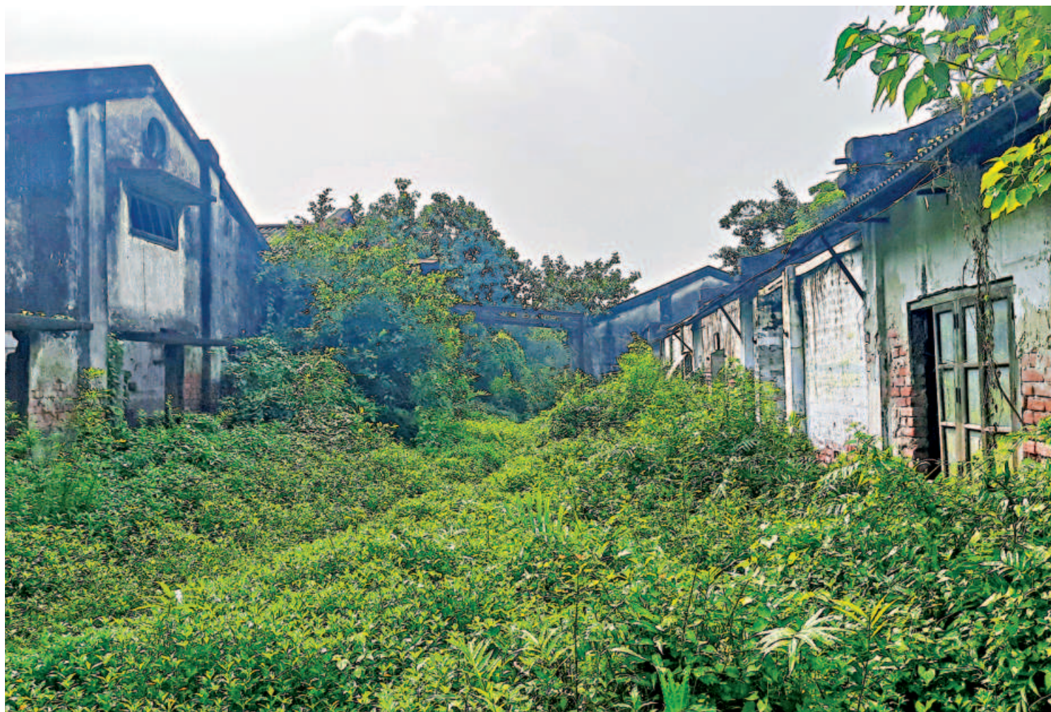
The Dada Match factory in Khulna city is seen covered in overgrowth as the grounds have remained vacant ever since the factory's closure in 2010. With virtually no initiatives having been taken to reopen the unit, most of the machinery and equipment have either been destroyed or stolen. The picture was taken recently.
