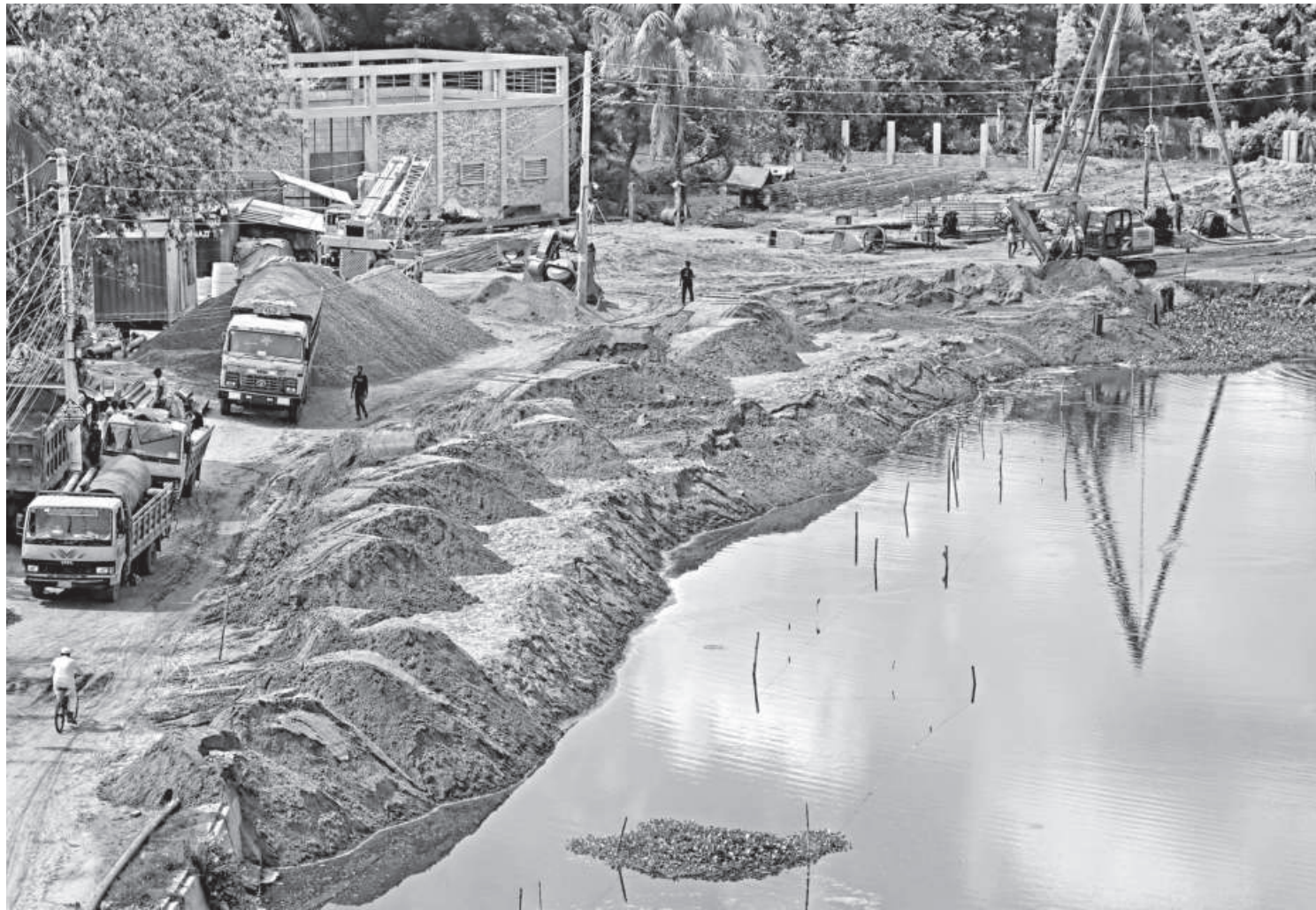
A part of the Nirala Dighi, the largest pond in Khulna city, is being filled up by the Khulna Development Authority for a road extension project.
