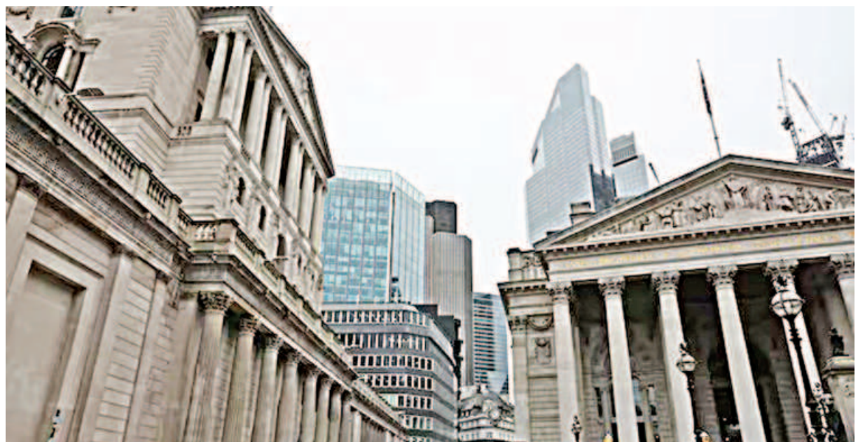
Road construction workers carry out work outside the Bank of England in London's financial district on February 13. PHOTO: REUTERS
