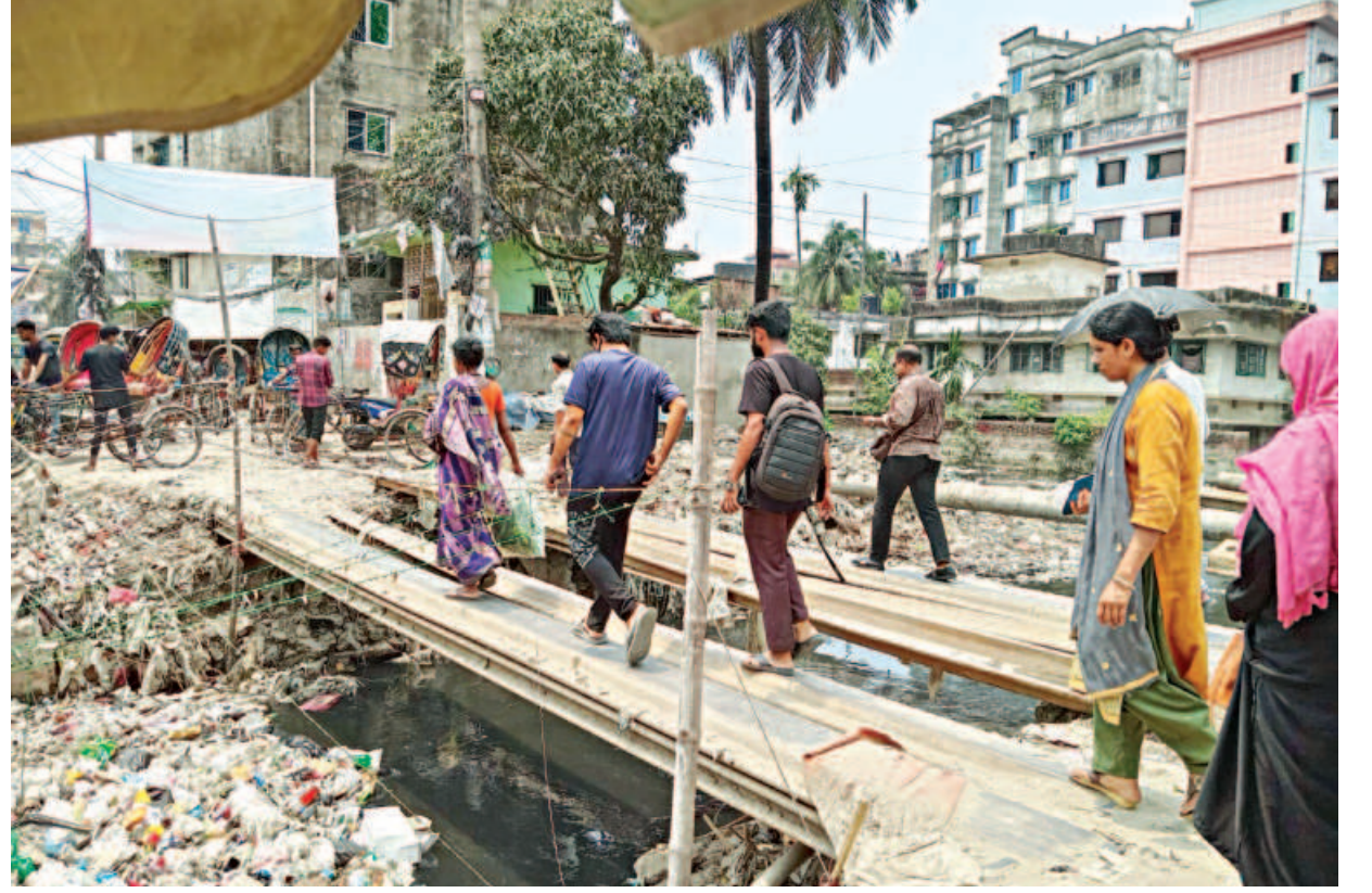
People cross this makeshift pathway, set up as part of ongoing works, in Chawkbazar Phooltala area. This temporary pathway not only makes it difficult for vehicles to cross, but also poses a risk to people as they can fall into the canal at anytime.
