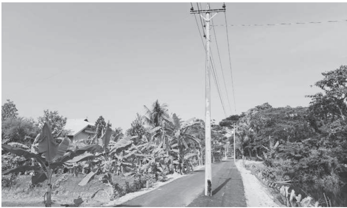
This electric pole is located on the middle of an approach road to a bridge on a canal in Char Montaj union of Patuakhali's Rangabali upazila. Despite construction work being completed six months back, the pole is yet to be removed. PHOTO: STAR
