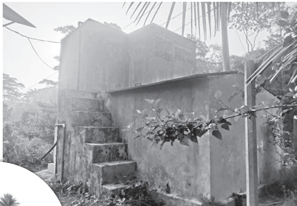
According to the Department of Public Health Engineering, the government agency alongside different voluntary organisations installed 2,799 pond sand filters in the upazilas since 1992-93. Of those, at least 1,326 are unusable at present.
