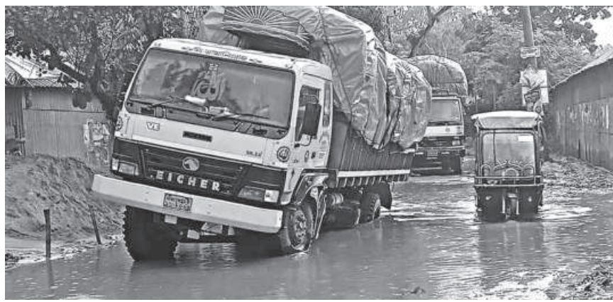
A truck remains stuck on Sakhipur-Sagardighi Road in Tangail after hitting a submerged pothole yesterday. The road has been in a dilapidated condition for a long time due to heavy traffic and lack of maintenance.
